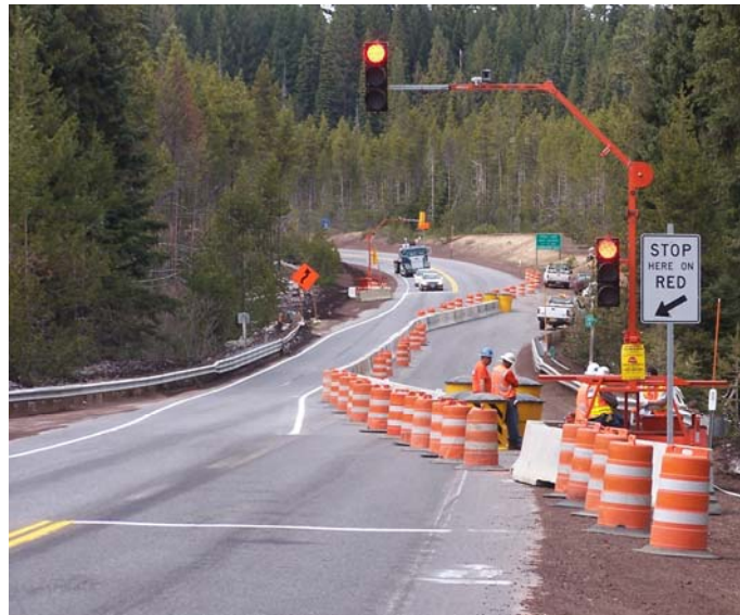
Figure 4-2: Example of a bi-directional work zone
