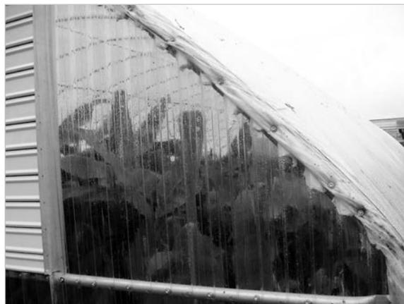
*Double polyethylene coverings and caulking air gaps help this greenhouse save energy.*
