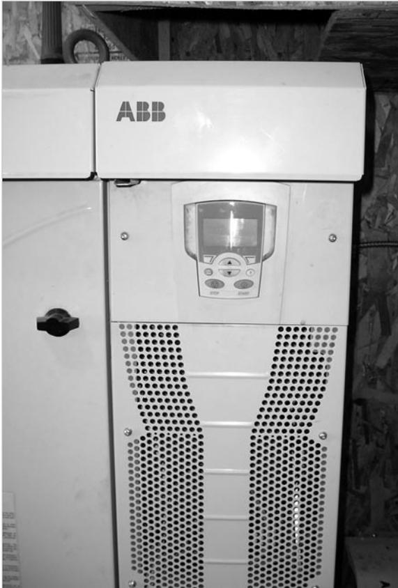
*This variable frequency drive ensures the irrigation pump will operate at the right speed for the size of the job, saving energy.*
