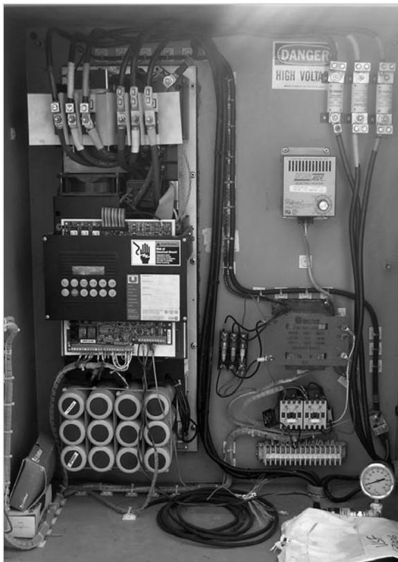
*This variable frequency drive ensures the irrigation pump will operate at the right speed for the size of the job, saving energy.*
