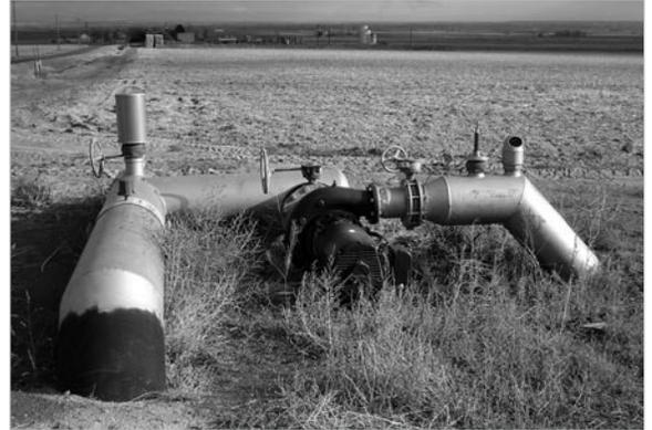
*A variable frequency drive controls the speed of this efficient pump in Malheur County, saving electricity.*
