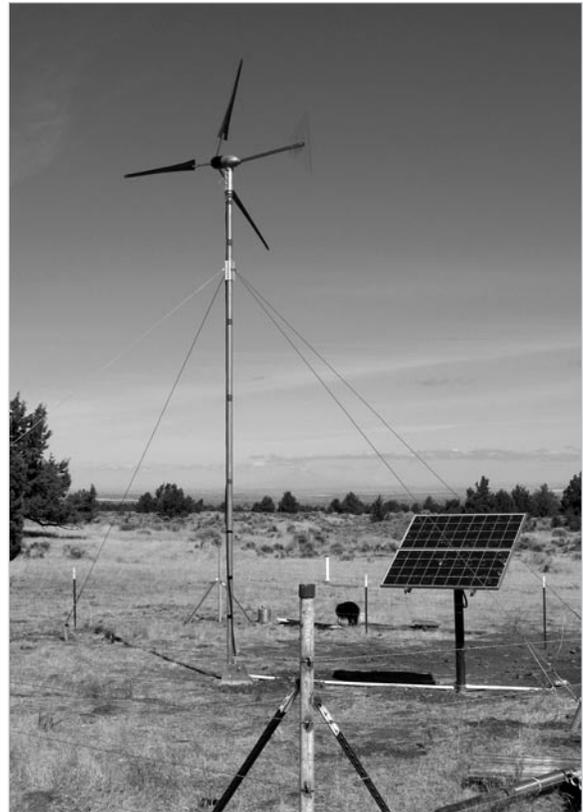
*This hybrid solar-wind system will power a pump for livestock watering in Sherman County*
