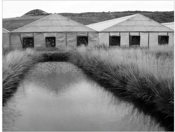
*Tailwater from the greenhouses on the Liskey farm heats these ponds, which are used to grow tropical fish.*
