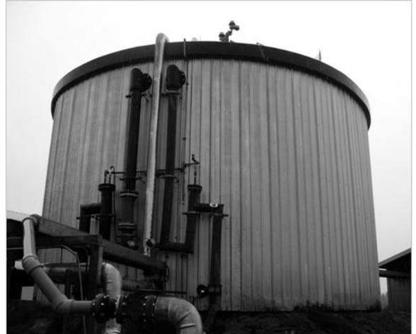
*Methane captured in this digester at Cal-gon Dairy in West Salem, Oregon, provides fuel to an engine that generates electricity.*
