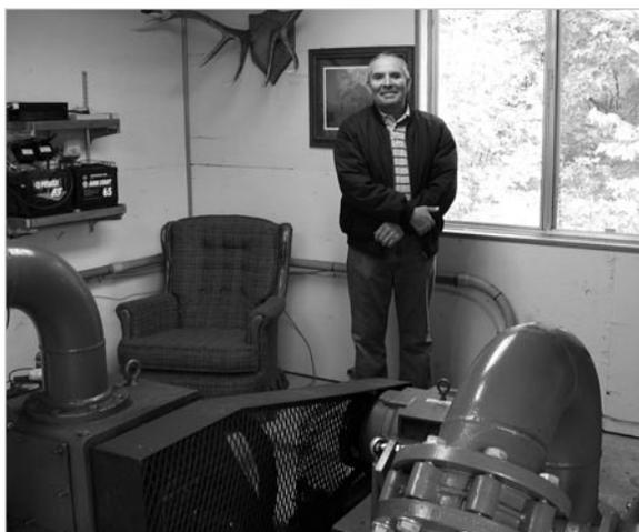
*Lucien Gunderman stands behind two turbines in the main hydroelectric facility. The turbines have a combined capacity of 30 kilowatts.*
