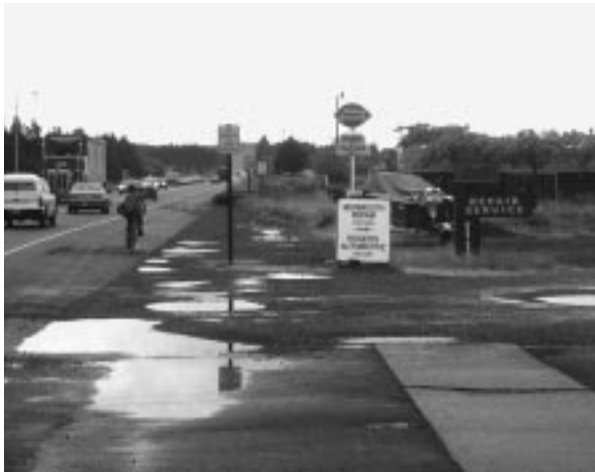
Sidewalk ends abruptly
