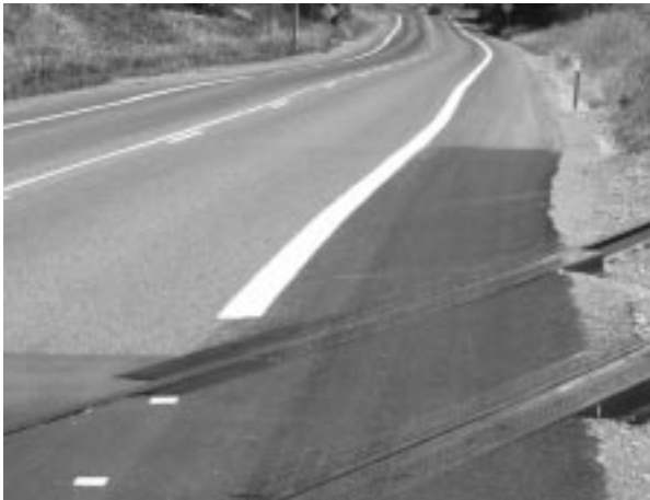
This rubberized crossing is smooth, with a narrow flange opening
