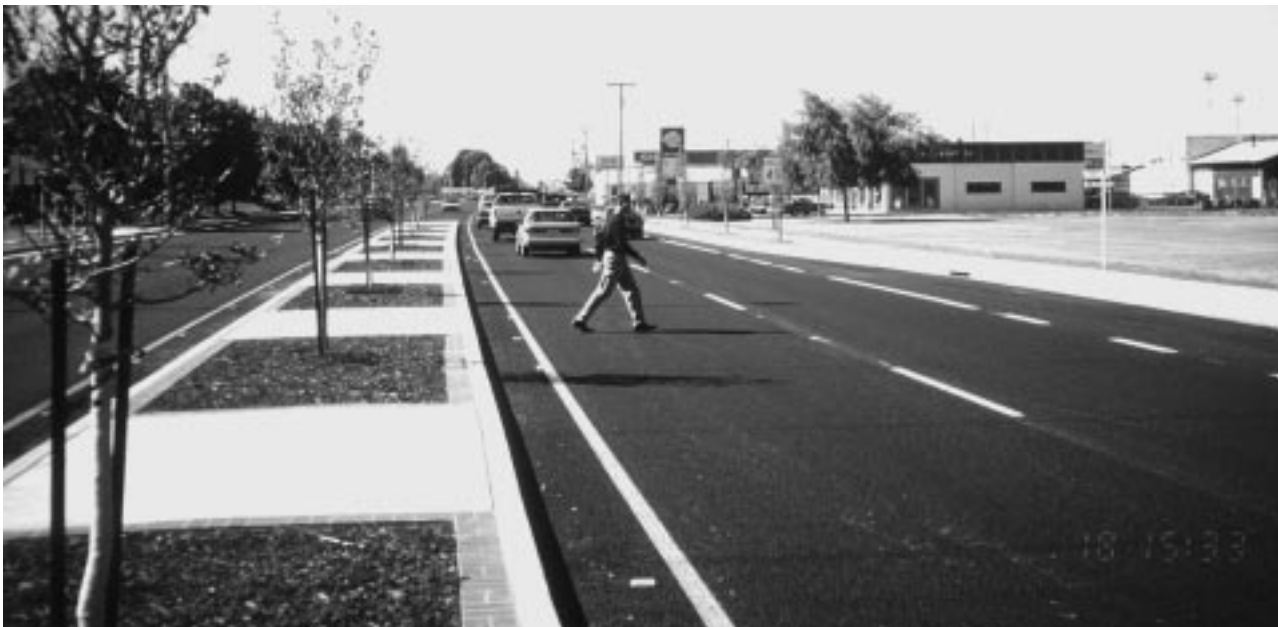
Median allows pedestrian to cross one direction of traffic at a time
