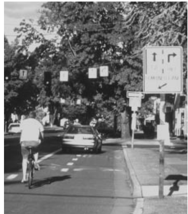
Combined right-turn lane and through bike lane
