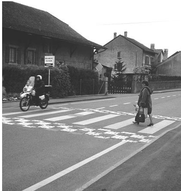
Raised and textured crosswalk (Switzerland)
