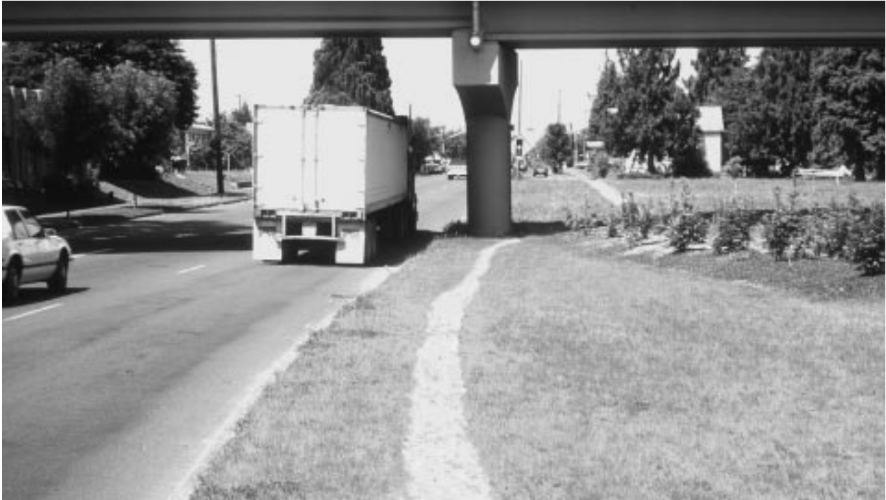
A beaten path indicates need for a sidewalk here
