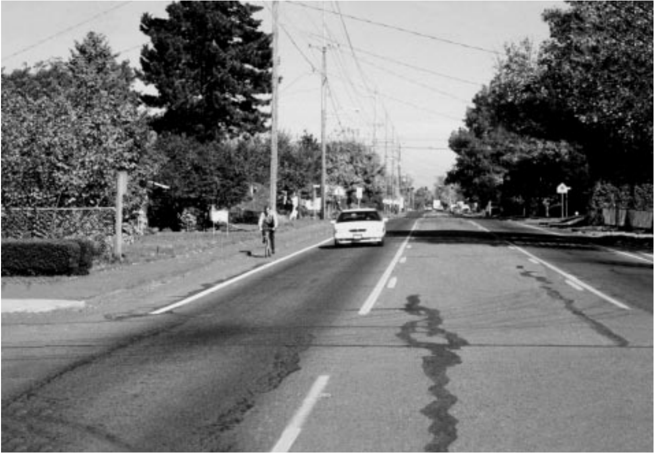
This street had four travel lanes before being reconfigured to three lanes and bike lanes
