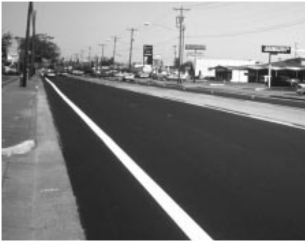
Thermo plastic stripes increase the visibility of bike lanes
