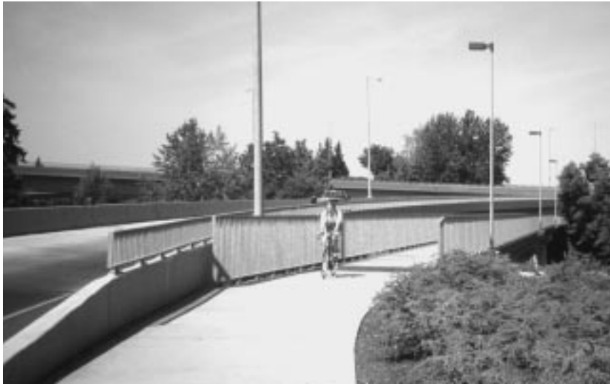
Structure with railing and illumination
