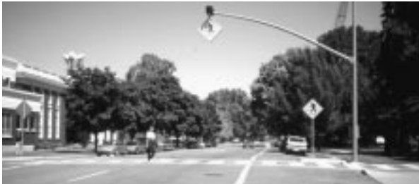
Pedestrian crossing signs
