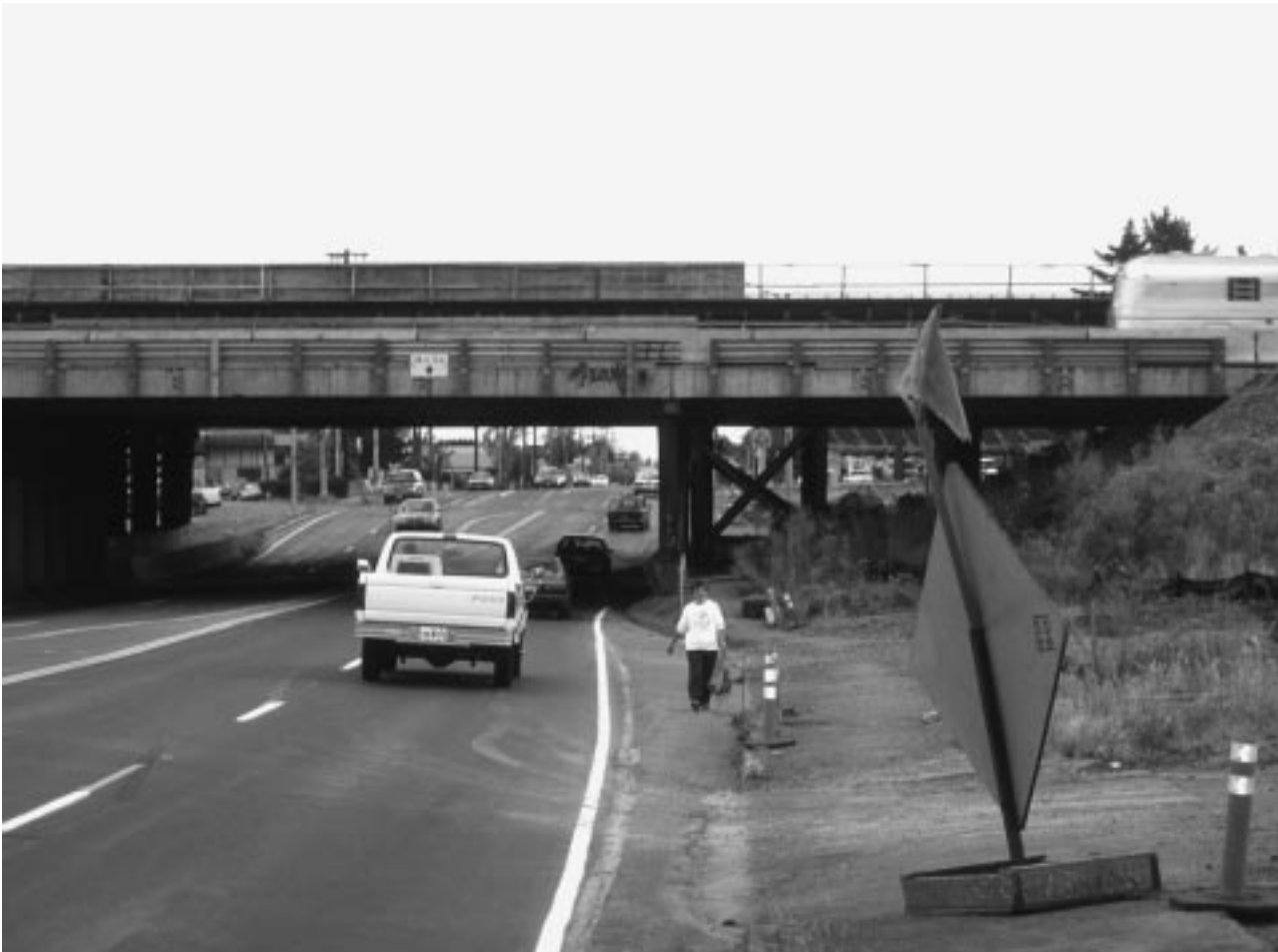
Pedestrians need access across freeway during construction
