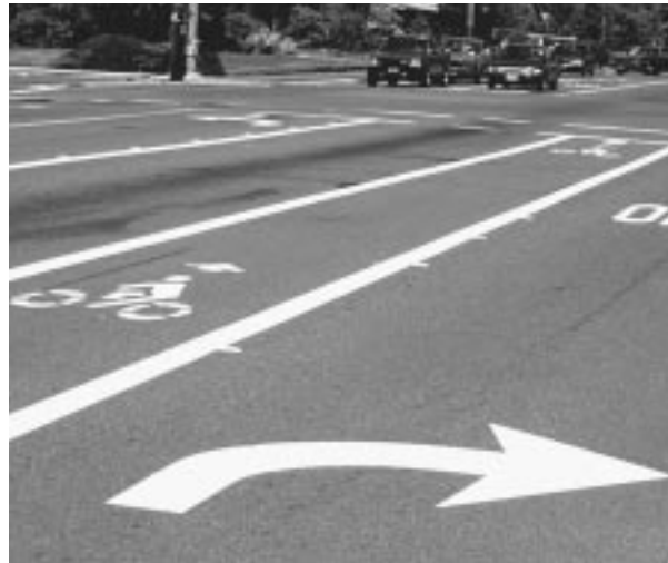
Raised pavement markings placed outside of the bike lane
