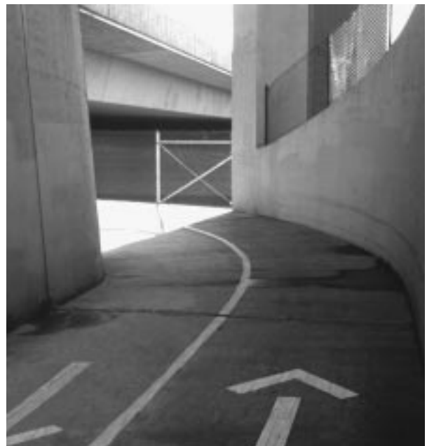
Striping and arrows in blind curve
