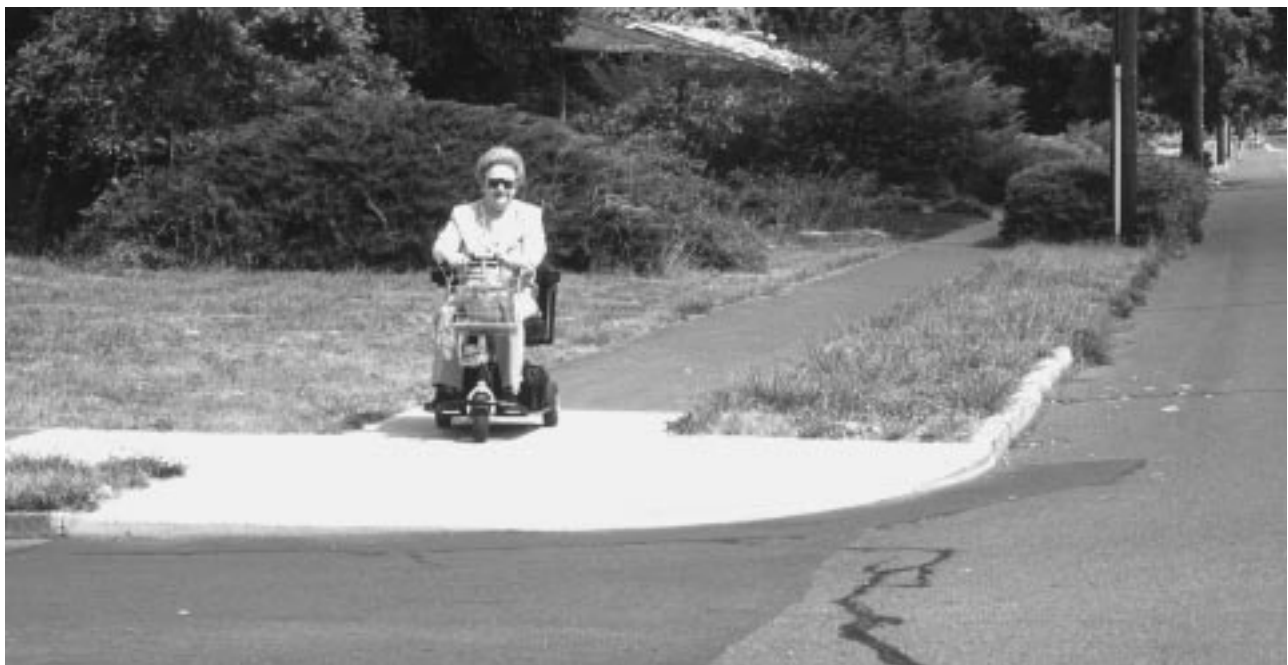
Curb-cut retrofit projects improve accessibility
