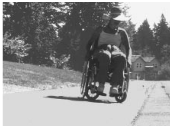
Sloping driveway creates difficulties for wheelchair users
