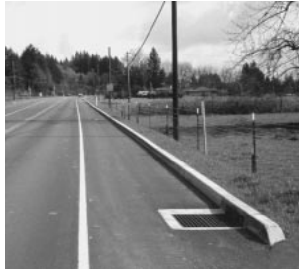
Well placed drainage grate
