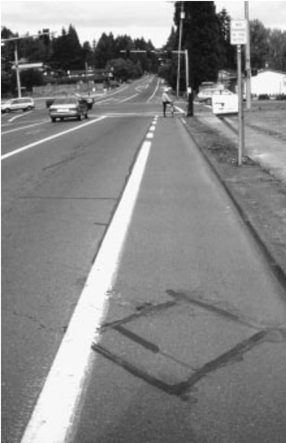
A loop detector in the bike lane should supplement push-button
