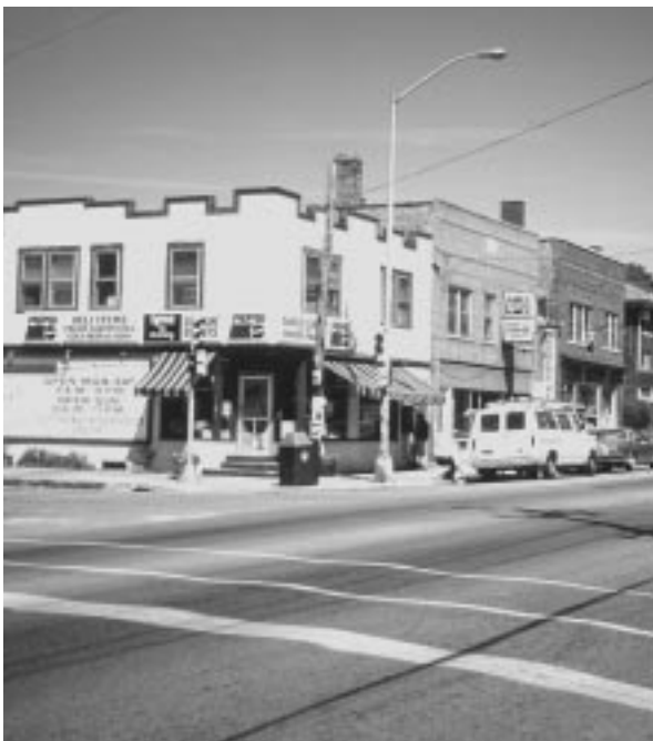
Traditional corner store is within walking distance of residential area
