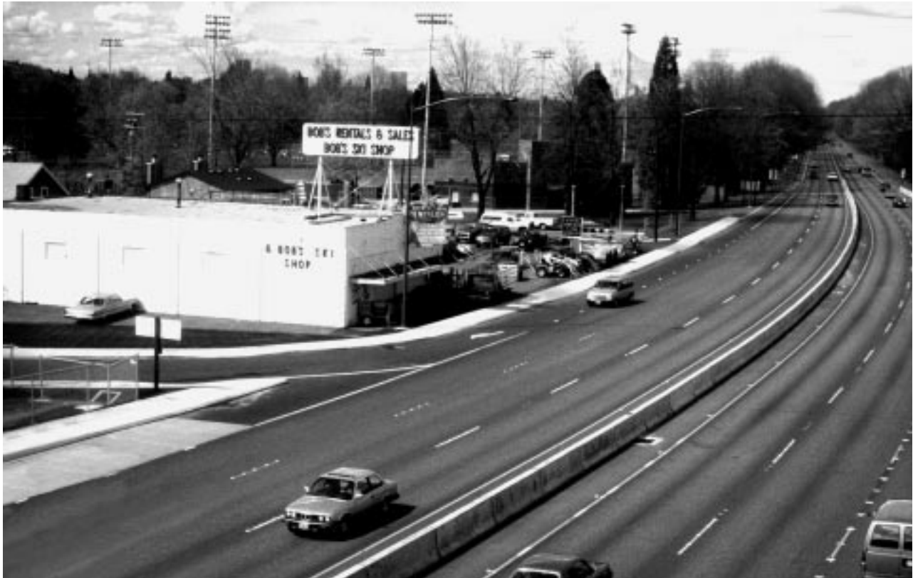
Concrete barrier in median prevents pedestrian crossing
