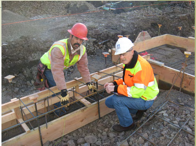
Smith and Fernando Guterrez discuss projection at the ends of the rebar slab dowels.
