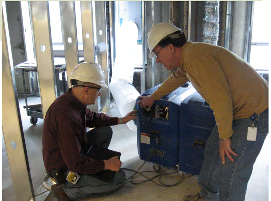
Pat Staed, a project superintendent, demonstrates the operation of an air scrubber at Medford's Rogue Valley Medical Center.
