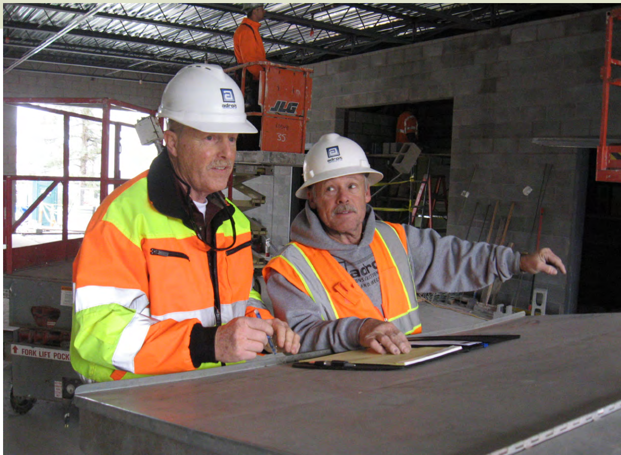
Smith (left) and Stan Robbins, a construction superintendent, review the safety plan at the Jackson County Jail Sally Port Project.
