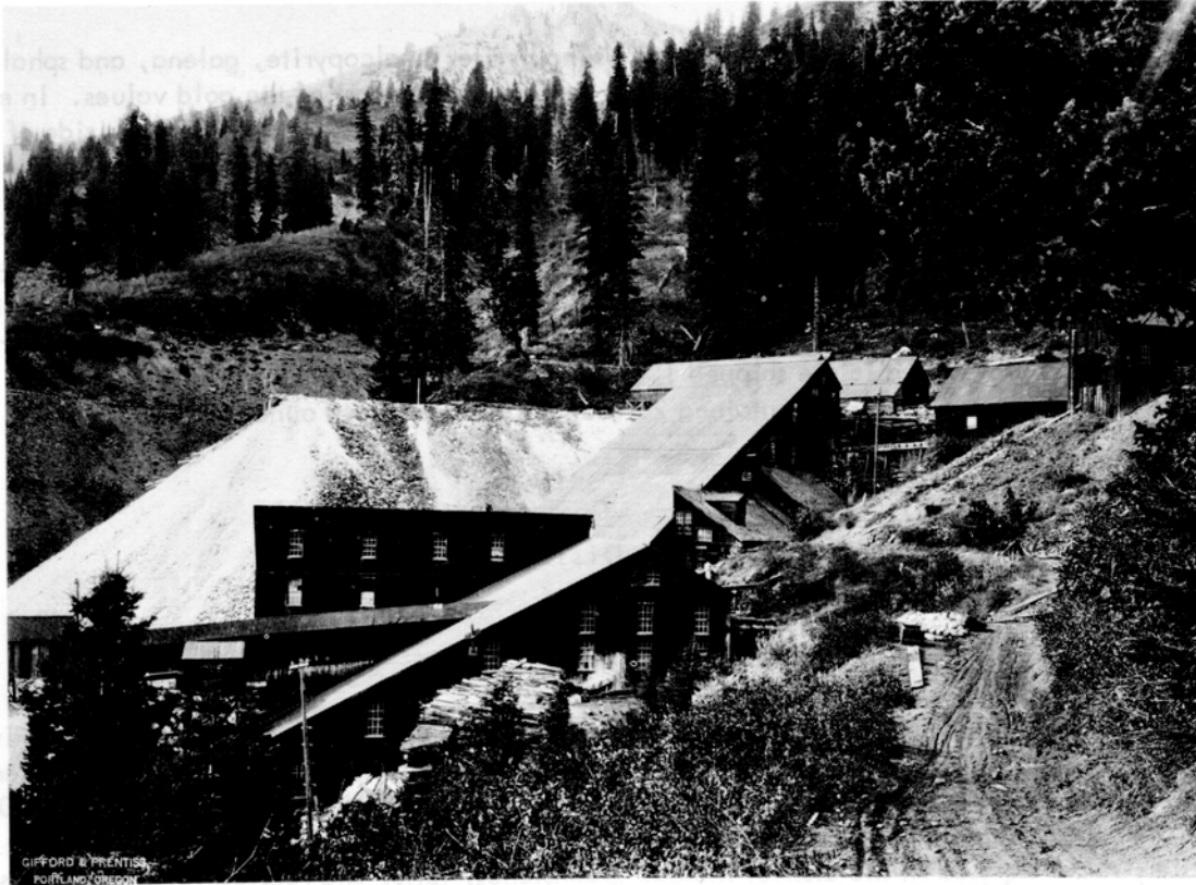
Figure 23. Union-Companion mill, Cornucopia district. Built at the portal of Clark tunnel in 1913.
