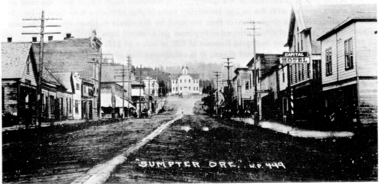
Figure 16. Main Street of Sumpter, Baker County, Oregon about 1914. Note board construction of street. (Photograph courtesy of Brooks Hawley.)
