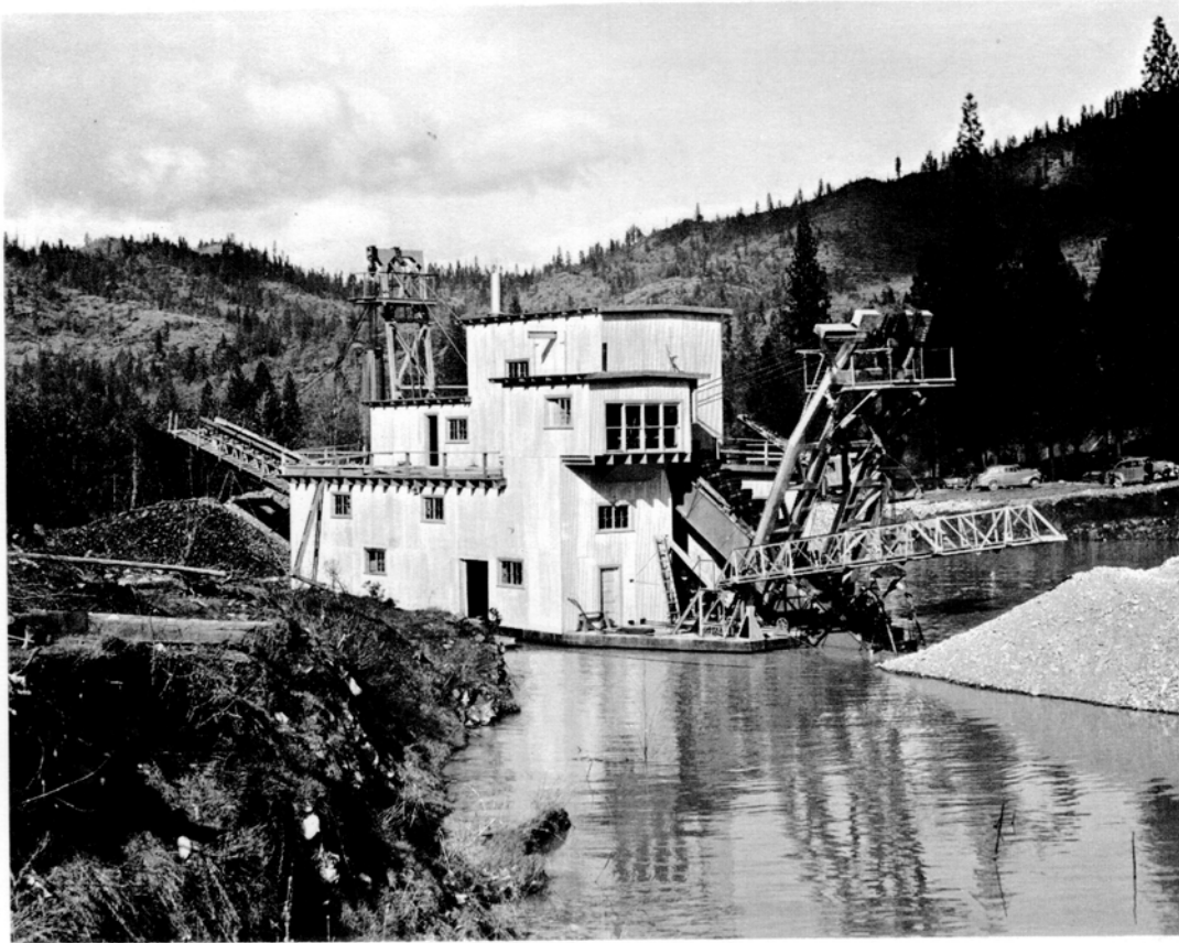
Figure 12-a. Murphy-Murray dredge on Footh Creek, Jackson County, in January 1941. Capacity 4000 cubic yards daily, electric powered, 67 buckets, of 3\frac{1}{2} -cubic-foot capacity; dug 20 feet below water line. Steel hull 81 by 37 by 6 feet, gantries, and superstructure.
