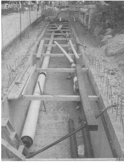
Figure 4. View of the tunnel under construction.
