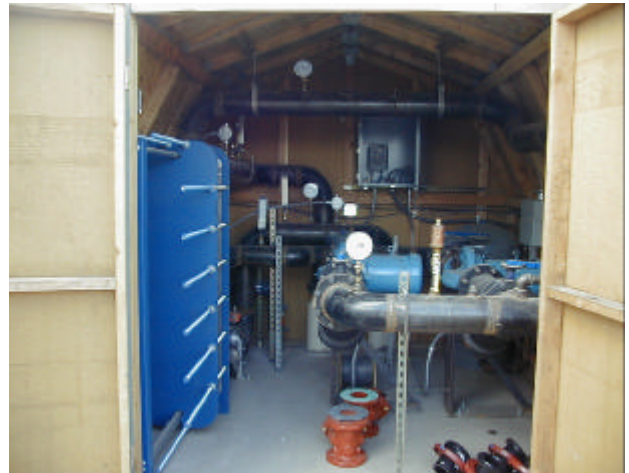
Figure 3. The main plate heat exchanger.
