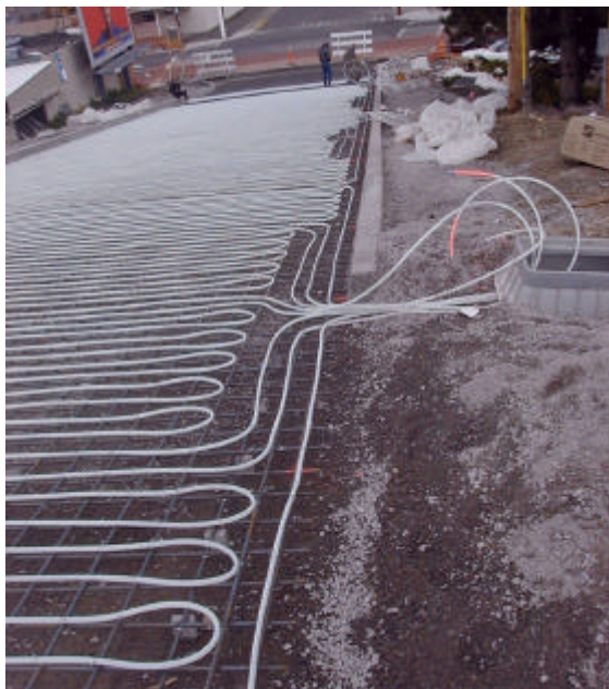
Figure 6. The approach road loops placed latitudinally.
