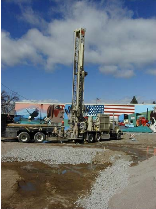
Figure 2. Photograph of drilling activities
