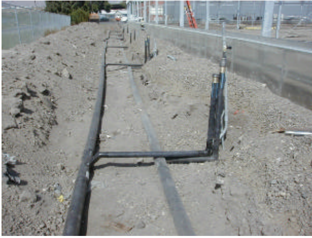
Figure 4. Secondary distribution system being installed for the new greenhouse.
