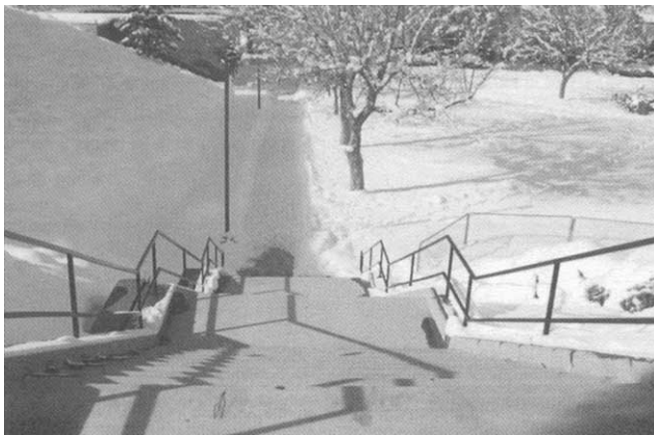
Figure 6. One of the stairwell leading to the College Union.
