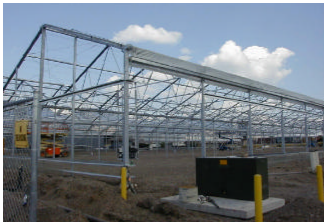
Figure 2. The second greenhouse under construction.
