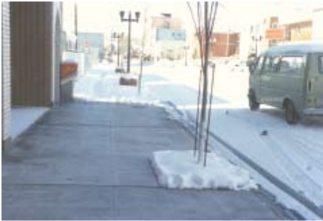
Photo 4: Geothermally Heated Sidewalk Snowmelt (Geo-Heat Center)
