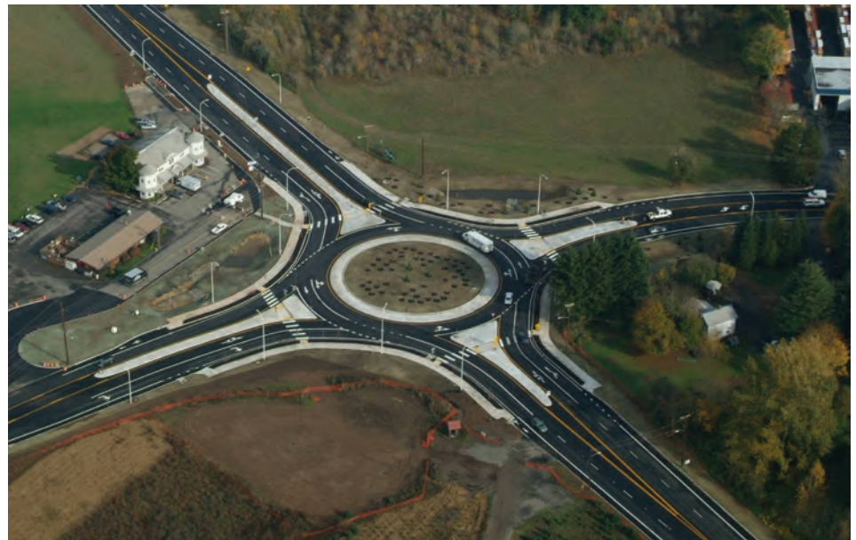
This roundabout at Borland and Stafford roads in Clackamas County was completed in October 2008. It's located just north of I-205 in the northwestern part of the county, east of Tualatin, south of Lake Oswego, and west of West Linn. Original plans called for a one-lane roundabout, but a 2006 study noted that 18,000 cars pass through the intersection daily and that number will only increase in the future. Traffic roadway engineers have found that roundabouts can carry 30% to 50% more vehicles than similar-sized signalized intersections.
