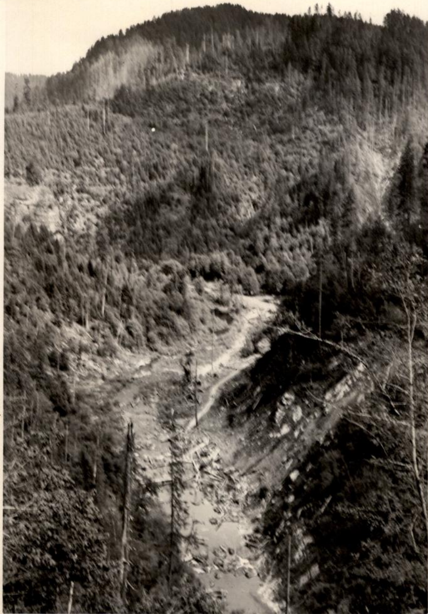
Fig. 41. Site of Coos River Boom Company's 1941 splash dam, RM 21.5. PUC File, State Archives
