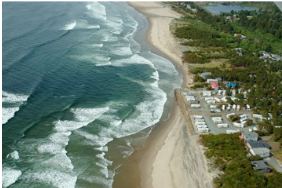
Figure 9. Ongoing shoreline retreat over the past decade in the Rockaway cell and localized hotspot erosion effects have resulted in substantial sections of the shore having to be rip-rapped in order to safeguard property. SLR expected over the next century and enhanced storms will almost certainly increase the risk of failure of such structures and the potential loss of homes and important infrastructure backing the beach (Photo courtesy of Mr. Don Best, 2009).
