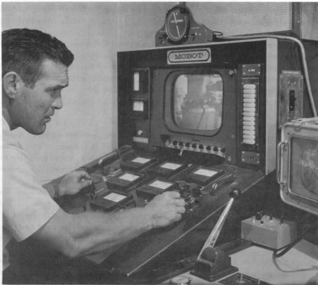
Figure 5. Electronic control panel for Shell's Mobot. Movements of the Mobot are monitored by use of closed-circuit television.
