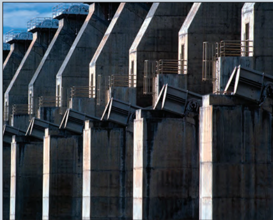
The Dalles Dam spillway
