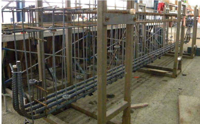
Figure 5.13: Example of reinforcing cage (T specimen shown)
