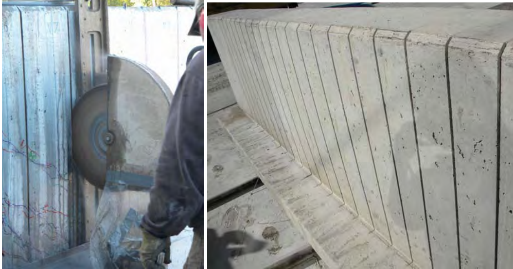
Figure 5.16: Typical vertical groove cutting technique and finished grooves
