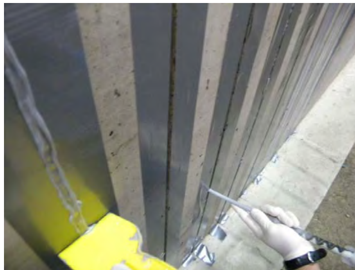
Figure 5.17: Epoxy placement over CFRP in saw cut grooves
