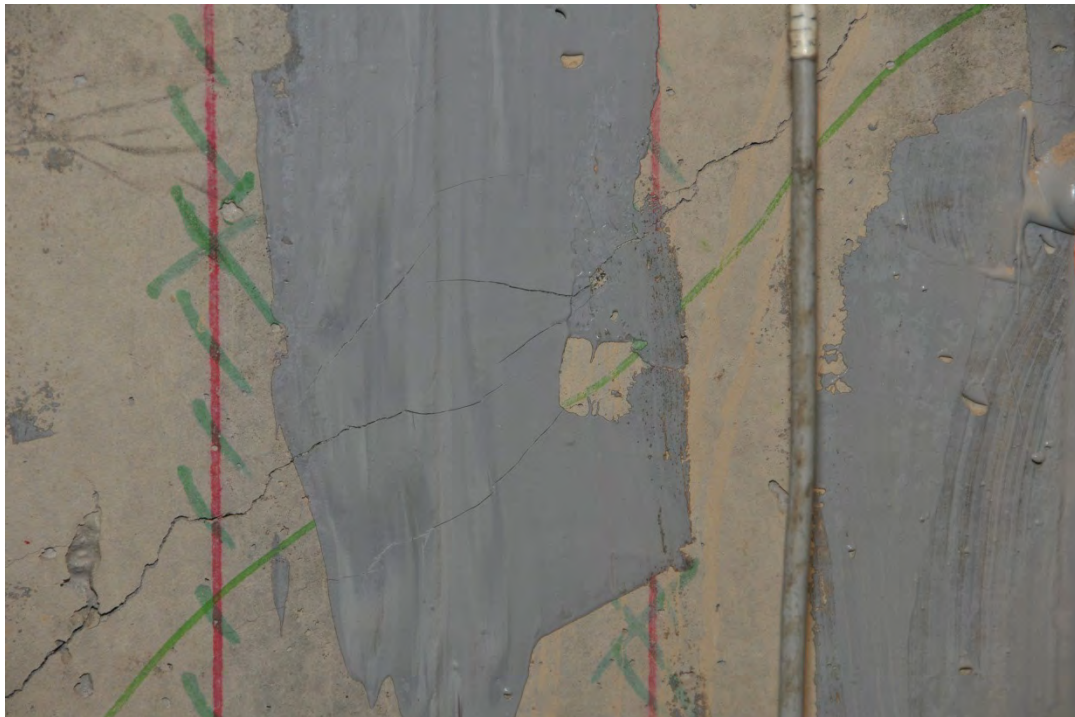
Figure 6.15: Example of crack feathering at NSM locations
