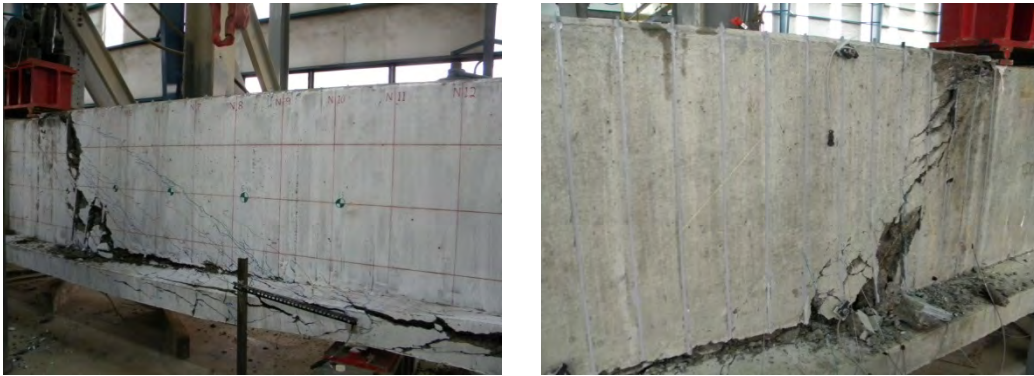
Figure 6.8: Specimen IT.7.22.6.FT/FTG at failure
