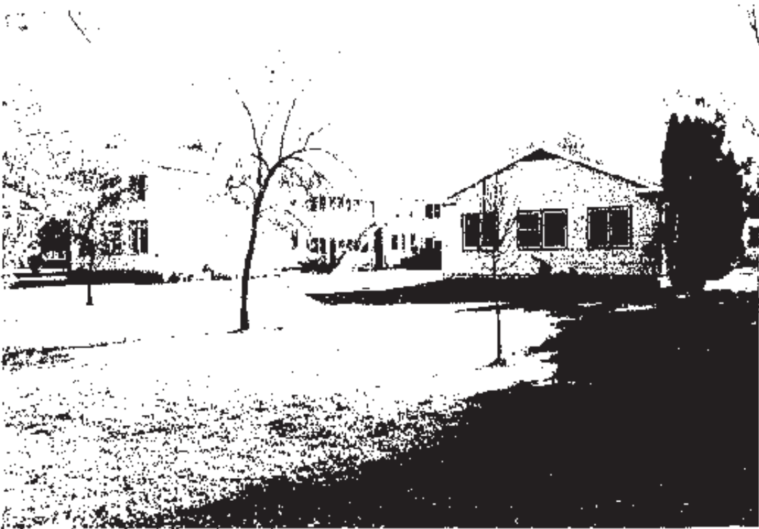
Wood Frame Barracks
