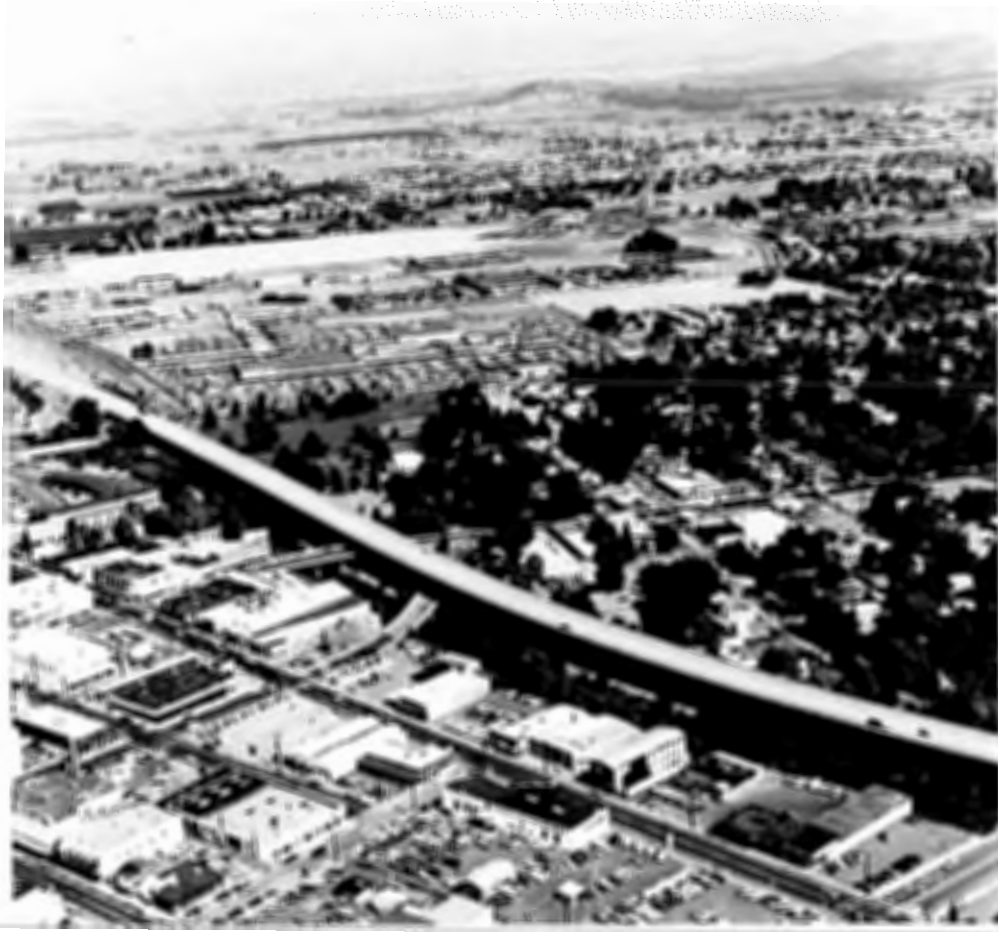
Figure 1.8. The Medford Viaduct, Looking NE over downtown, c. 1963 Source: ODOT Archive
