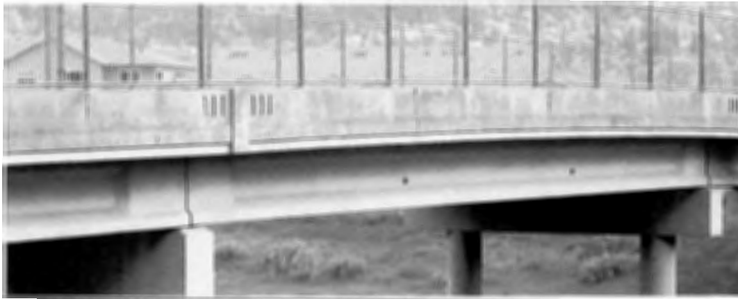
Figure 2.22. Typical Pre-Cast I-Beam with "Panel" Sides, Mountain Ave Overpass, I-5 Jackson County, Bridge #8739, 1963 Source: Author Photograph, May 2003
