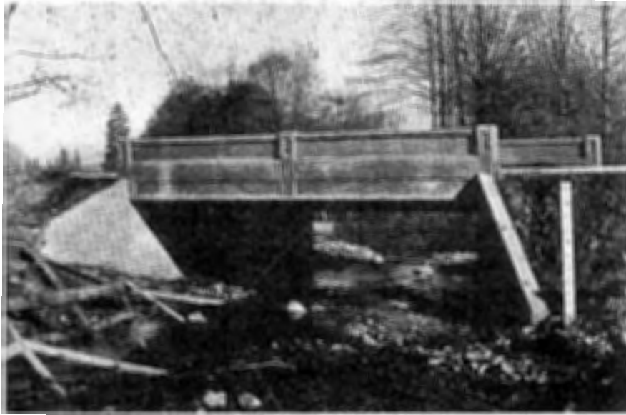
Figure 1.9. “Type of Concrete Bridge Erected Along Pacific Highway in Jackson County” Source: Medford Mail Tribune , 1-January-1915
