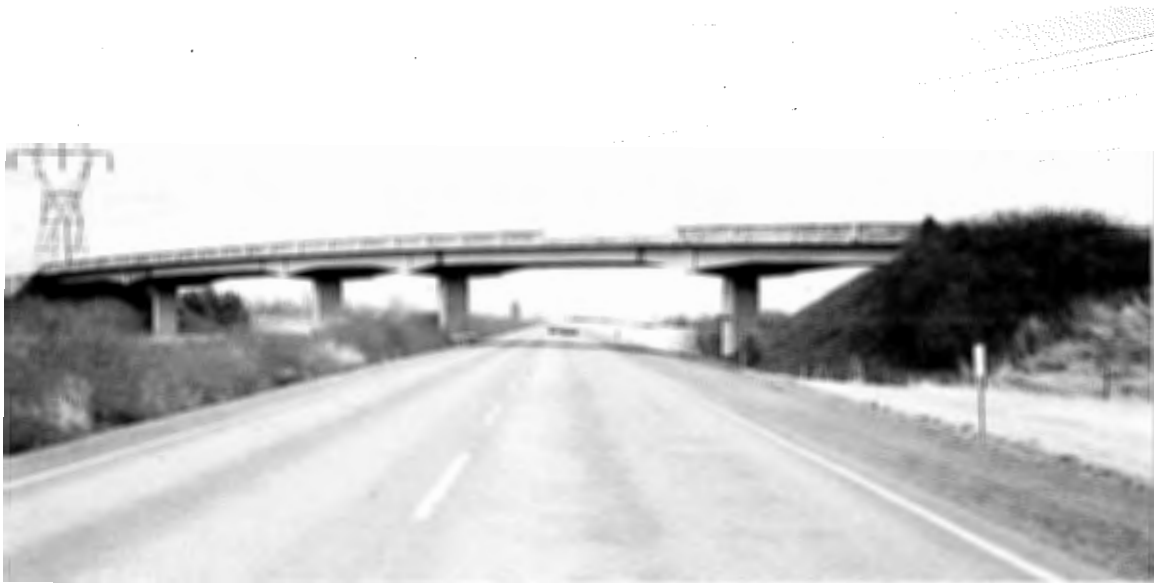
Figure 4.1. Gervais Road Undercrossing, Northbound Interstate 5 Source: ODOT General Files Photo, January 1971
