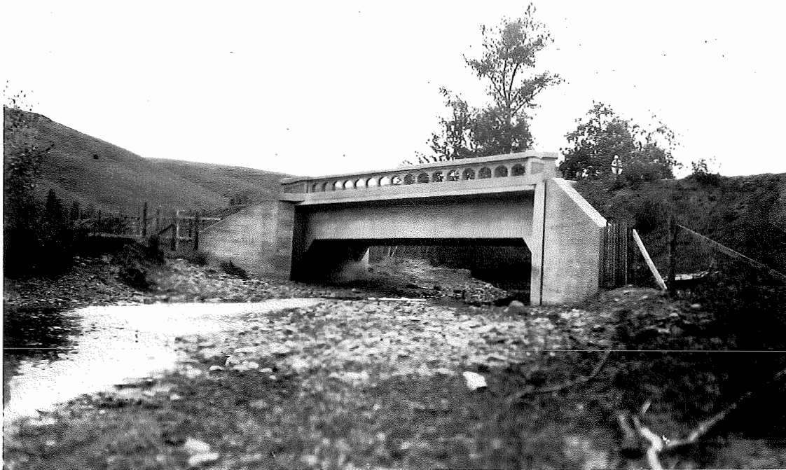
Figure 1.22. Perry Overcrossing, Baker-Unity Highway, Photo Date 1939 Source: ODOT Archive
