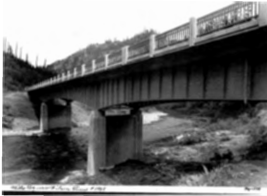
Figure 2.25. Mills Bridge, over Wilson River, (Bridge #1868) Source: ODOT Archive
