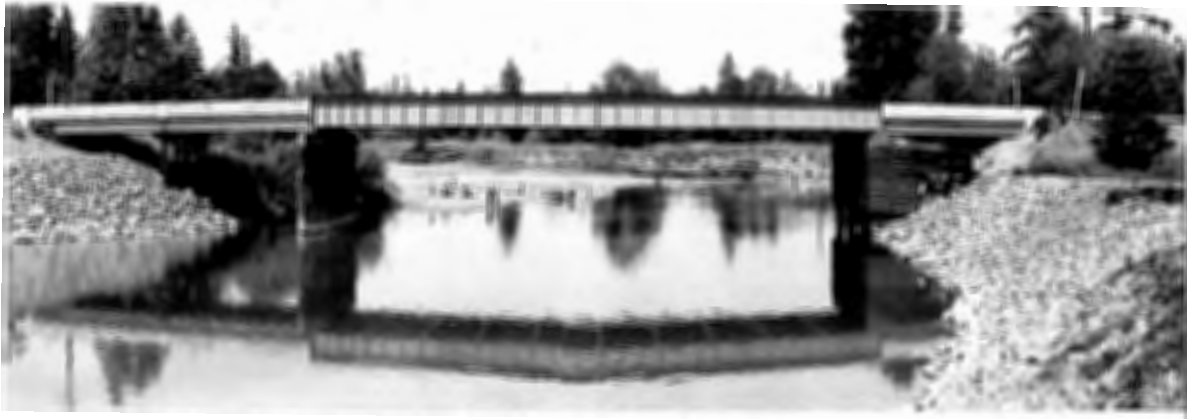
Figure 1.6. Pudding River (Red) Bridge on Arndt Road, Bridge No. 6521, c. 1950s (presumed razed) Source: ODOT Archive
