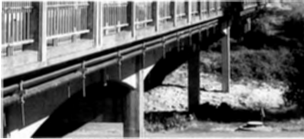
Figure 2.21. Haunched Girder, Isaac Constant (Bear Creek) Bridge (Eastbound) Jackson County, Bridge #697, 1948 Source: Author Photograph, November 2002
