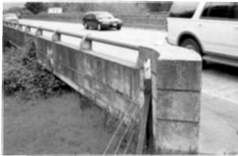
Figure 2.10. One-Pipe Parapet Rail, Bear Creek/I-5 Bridge #8890N, 1962 Source: Author Photograph, May 2003
