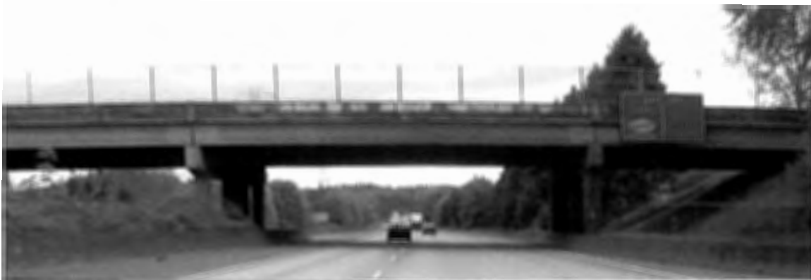
Figure 1.19. Typical Pre-cast I-Beam Overpass, Interstate 5, Lane County, OR Source: Author Photograph, May 2002
