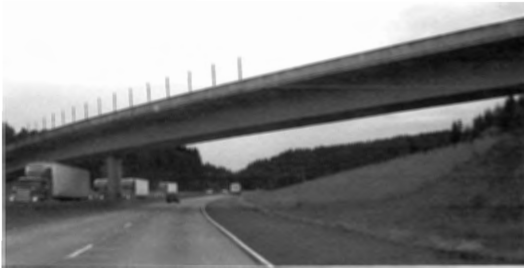
Figure 1.21. Box Girder Overpass on Interstate 5, Douglas County Source: Author Photograph, May 2002
