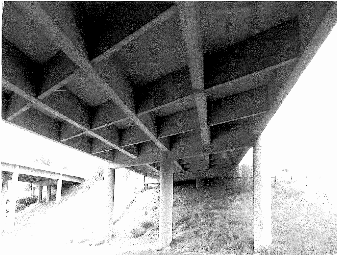
Figure 2.27. Round Section Piers, Bridge No. 8738N Interstate 5 over Eagle Mill Road, Jackson Cty, 1962 Source: Author Photograph, May 2002
