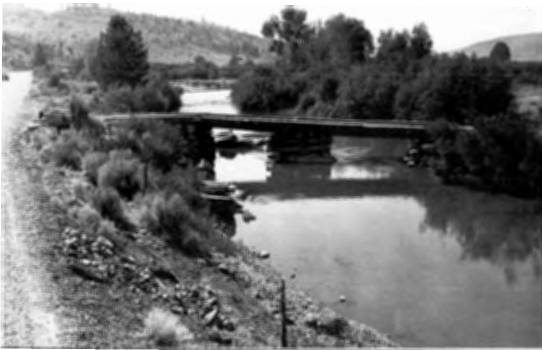
Figure 1.3. Log bridge, Klamath-Falls-Lakeview Highway over the Sprague River, 1930 Source: ODOT Archive
