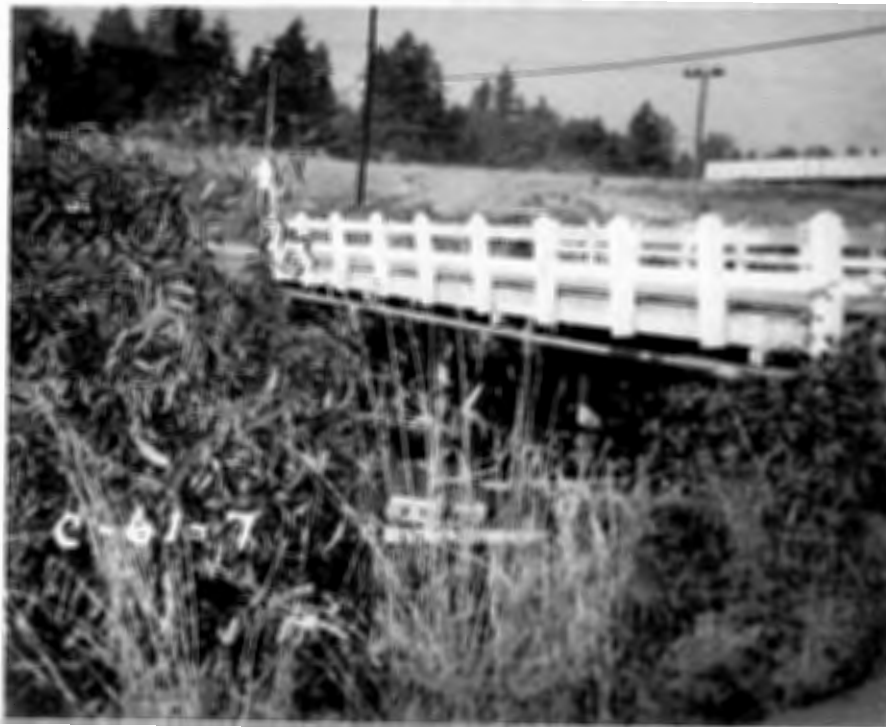
Mill Creek Bridge on Mill Creek Rd., in Milwaukie 10/13/61
