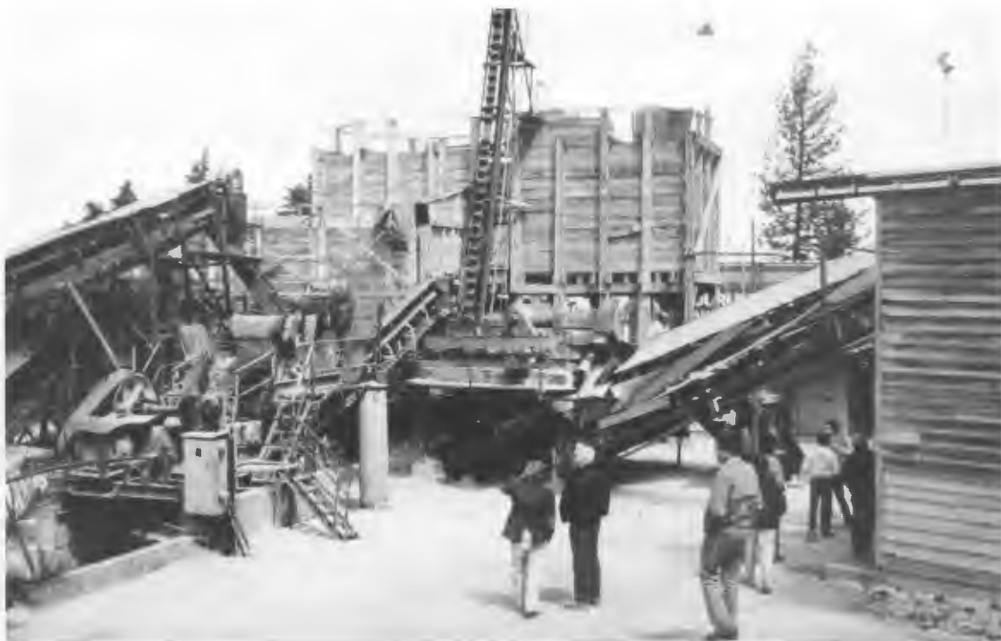
Figure 15. Crushing and screening plant of Central Oregon Pumice Company.
