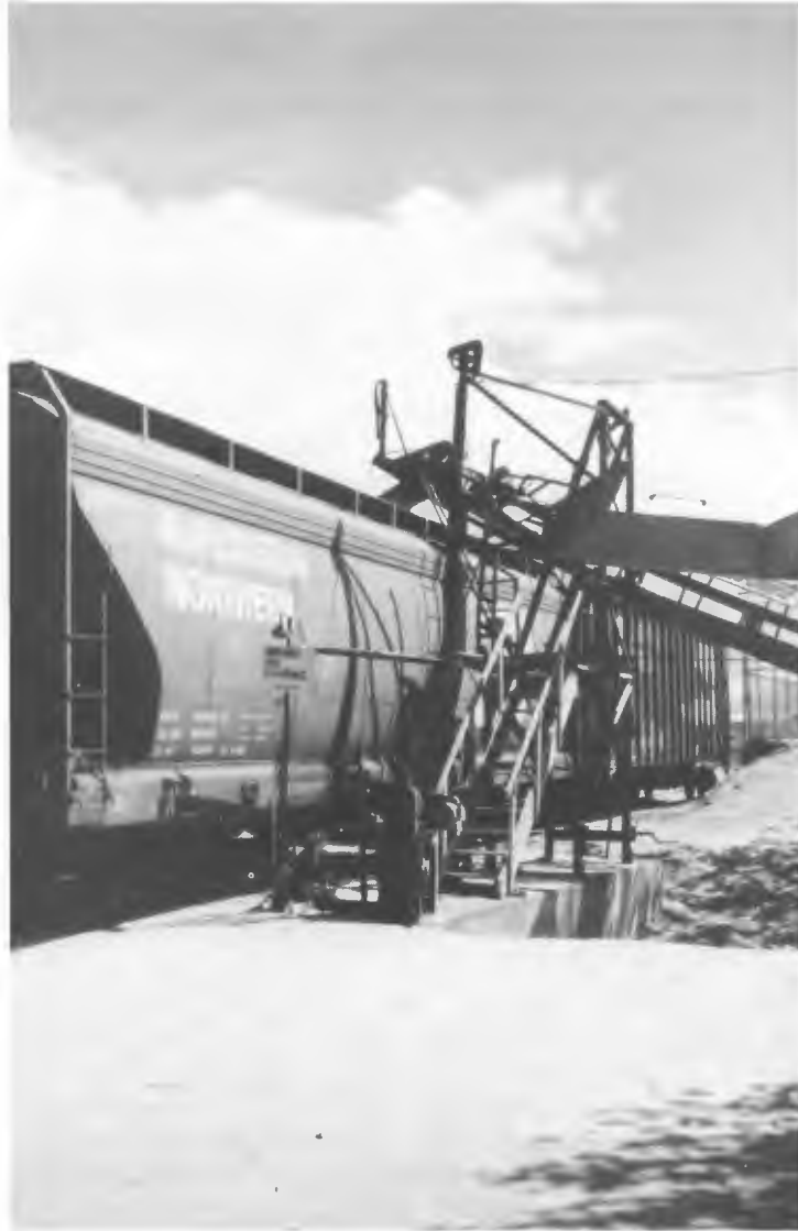
Figure 16. Rail-car loading facility, Central Oregon Pumice Company.
